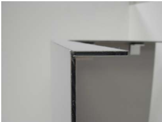
Curved Corner Panel Using a Cope
